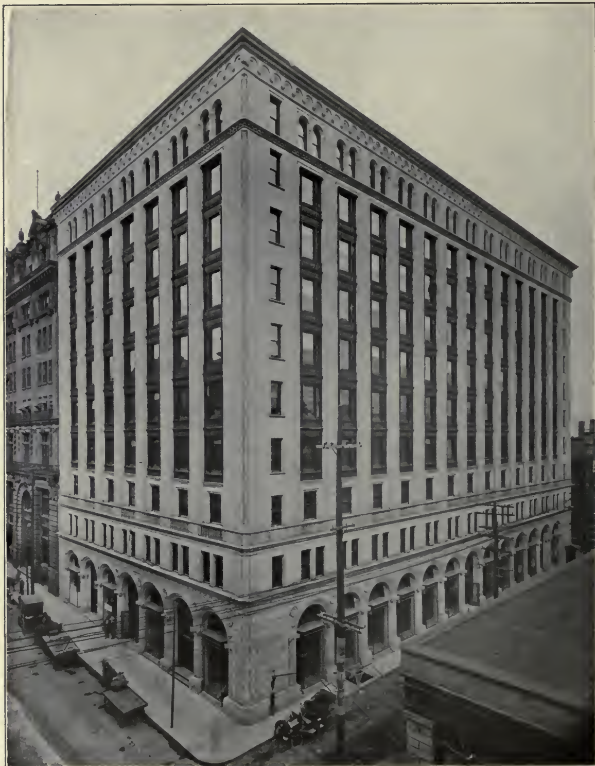
Transportation Building. Erected in 1912. Said to be the largest office building in the British Empire. It is the home of many large business and professional interests in Montreal.
